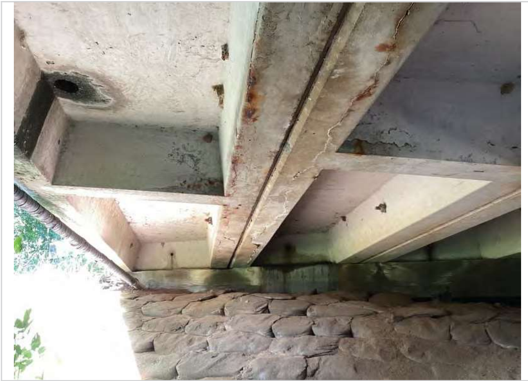
Span 3 Pre Cast Concrete Slabs A & B impending Spall
