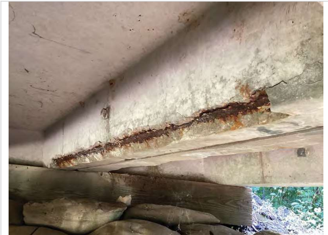
Span #1 PCCS "B" spall to steel
