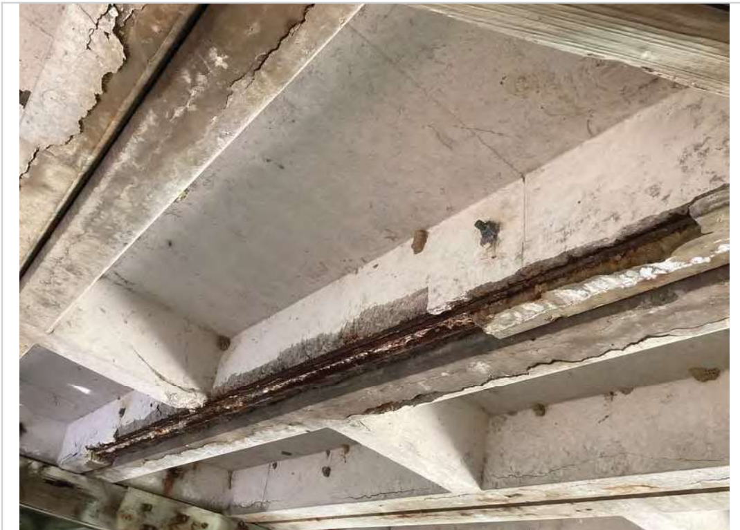
Span #2 PCCS "D" spall to steel
