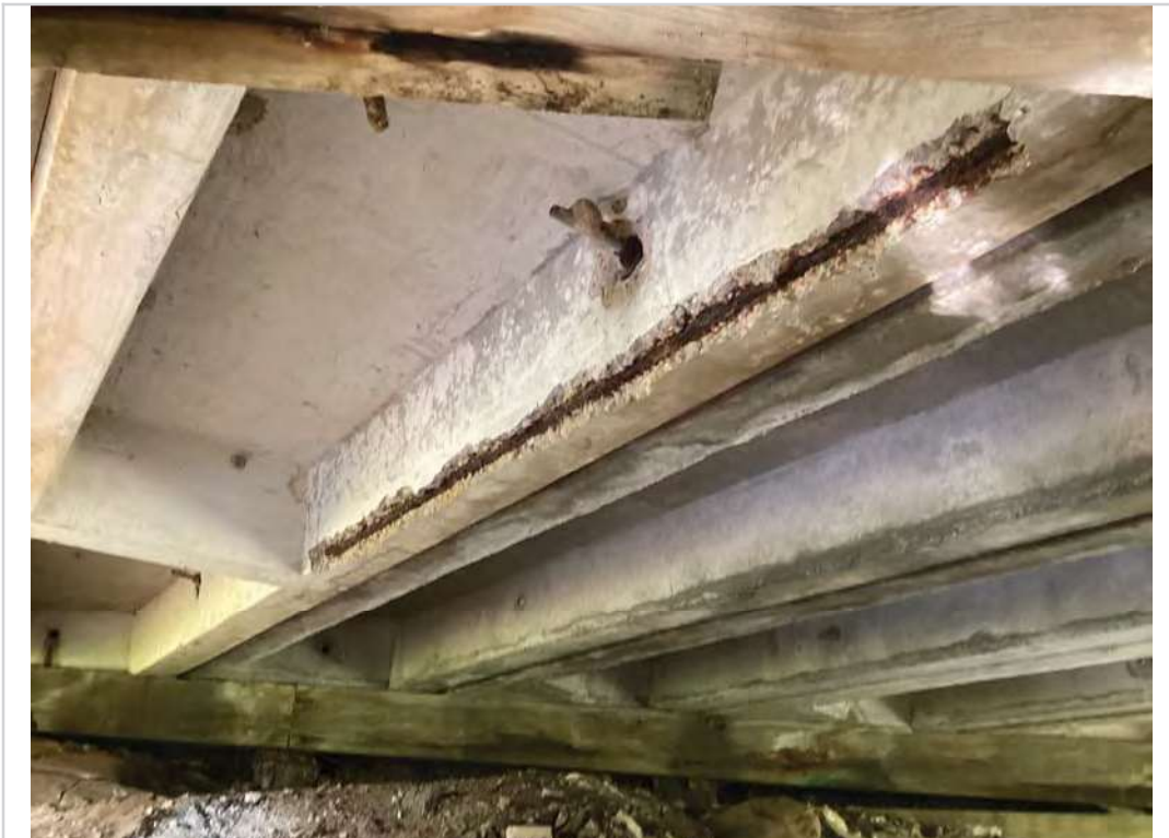
Span 3 Pre Cast Concrete Slab C spalled to steel on Right leg
