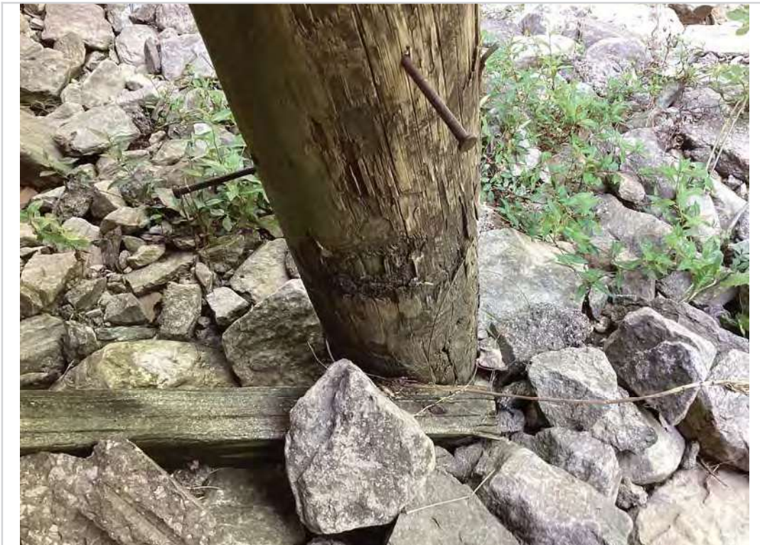
Bent # 1 Pile E, shakes
