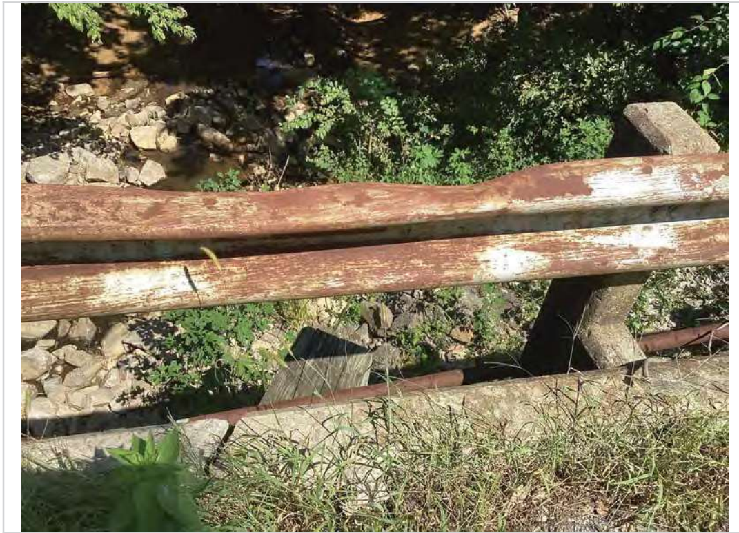
Span 1 rail damage
