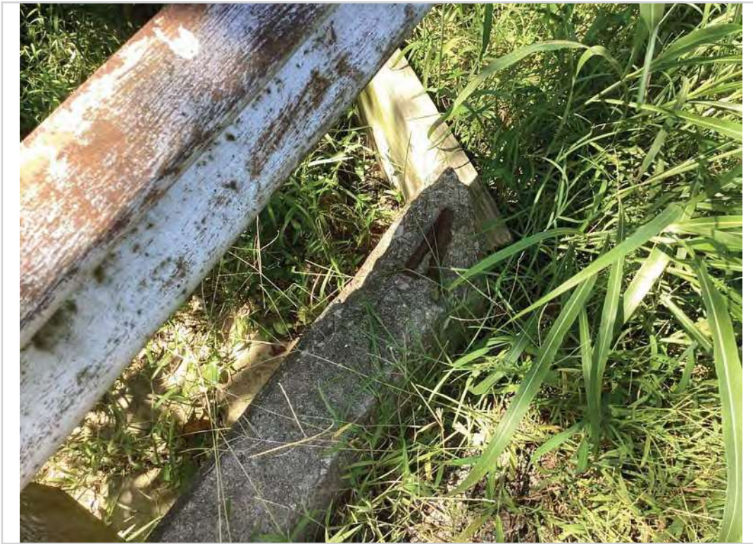
Span 3 curb spall to steel
