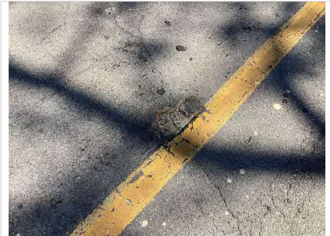
Span 2 spall
