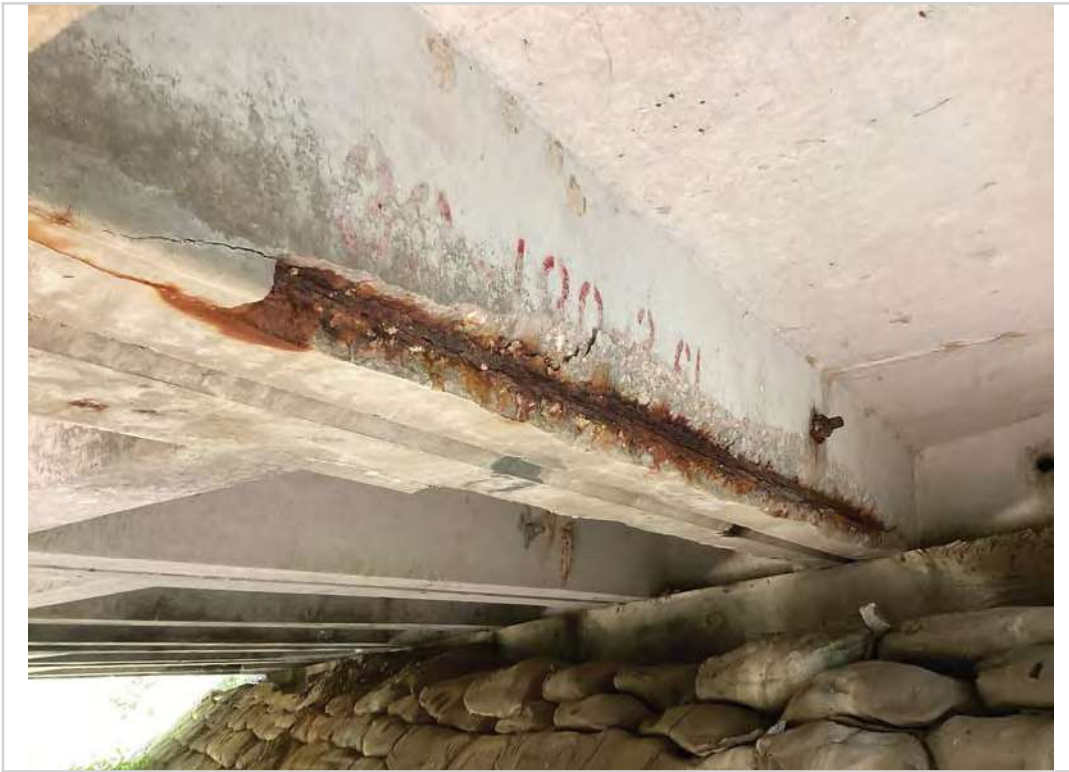
Span #1 PCCS "A" spall to steel
