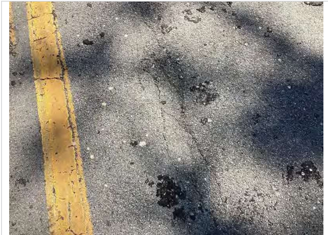
Span 1 crack
